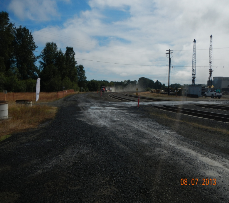
Photo 1. Unknown levee realignment adjacent to the PGE Port Westward Unit II natural gas power generating plant
