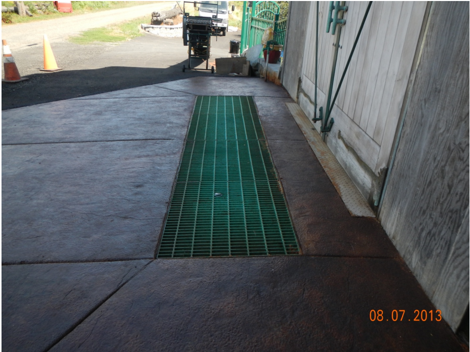
Photo 5. Surface water drainage structures of unknown construction installed within the levee prism.
